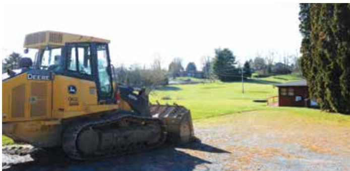
DELIVERY OF THE FIRST EXCAVATOR TO THE PROPERTY
