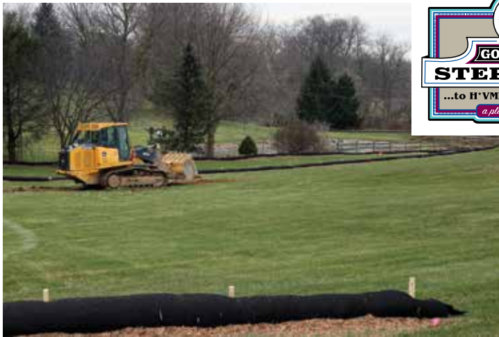
EXCAVATOR ON THE EASTERN SIDE OF THE SITE
