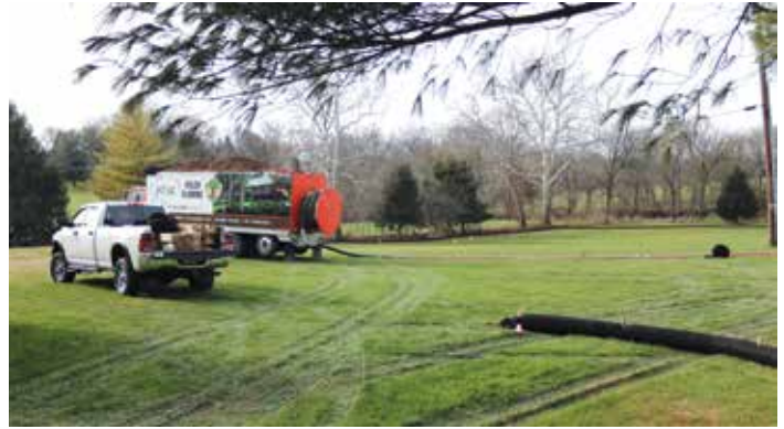
FILLING THE SILT SOCKS ALL OVER THE PROPERTY
