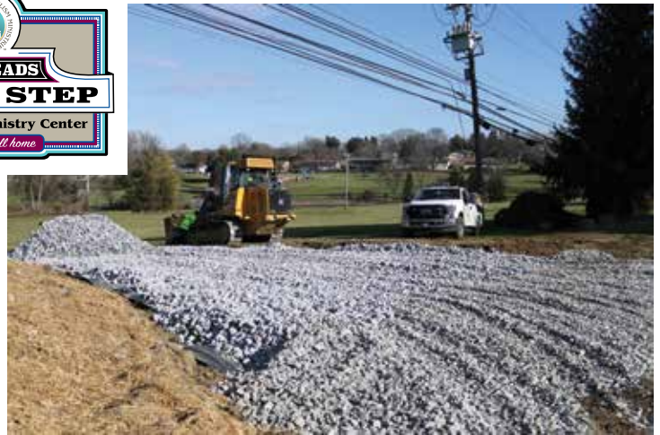
WESTERN ENTRANCE DRIVE WAY
